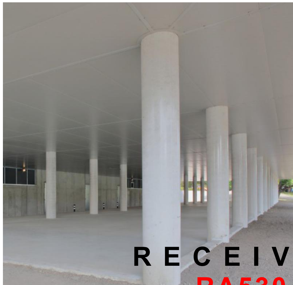
CONCRETE EXTERIOR COLUMNS
