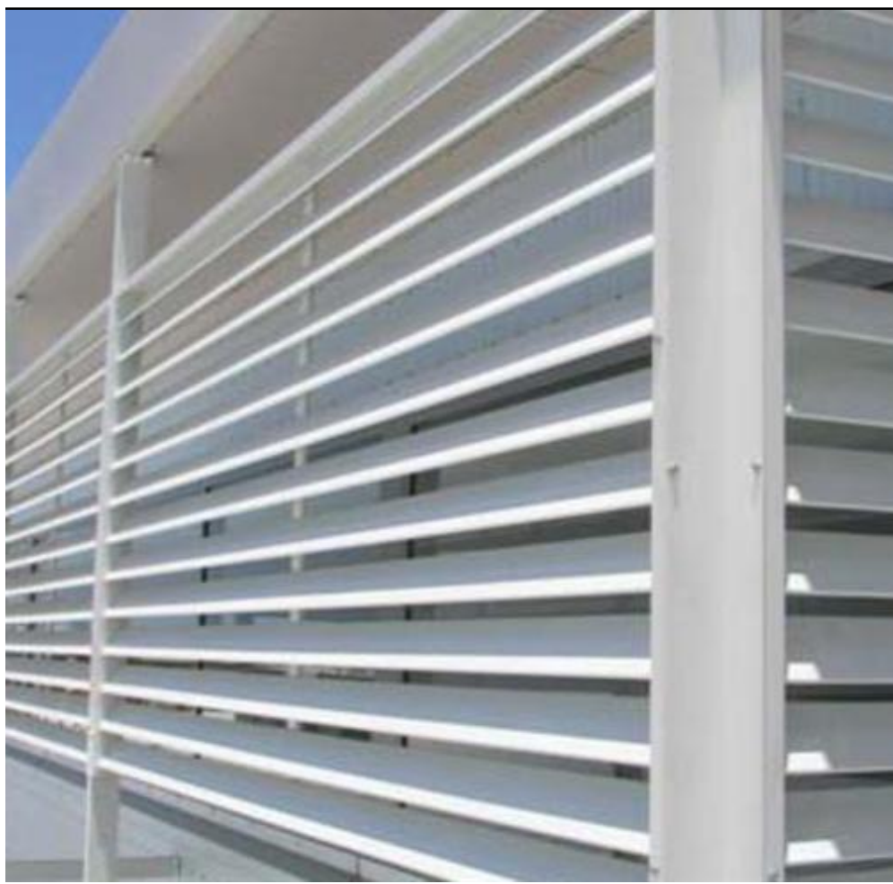
ROOF HVAC SCREEN
