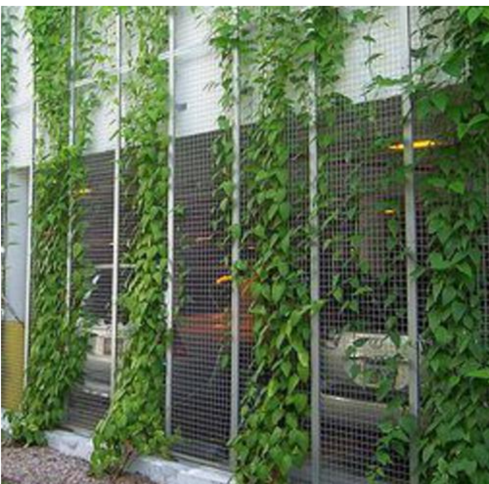
PARKING GARAGE GREEN WALL STUCTURAL SUPPORT
